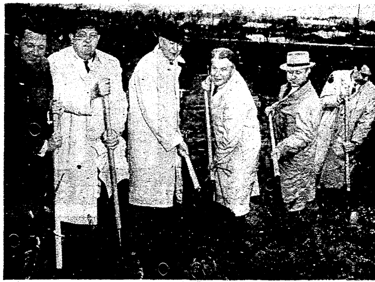
GROUND BROKEN—Ground was broken on the Eastern State College campus at Richmond yesterday for building projects costing more than $3,000,000. Participating were, from left, Robert Matthews, state finance commissioner; Dr. Robert R. Martin, Eastern president; Judge Thomas B. McGregor, Frankfort, member of the board of regents; Gov. Bert Combs, Wendell P. Butler, state superintendent of public instruction, and William Seent, state revenue commissioner.
